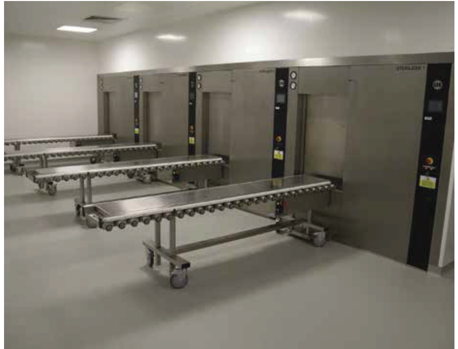
The LTE Scientific 42cu ft sterilisers were sized to suit the width of the building
